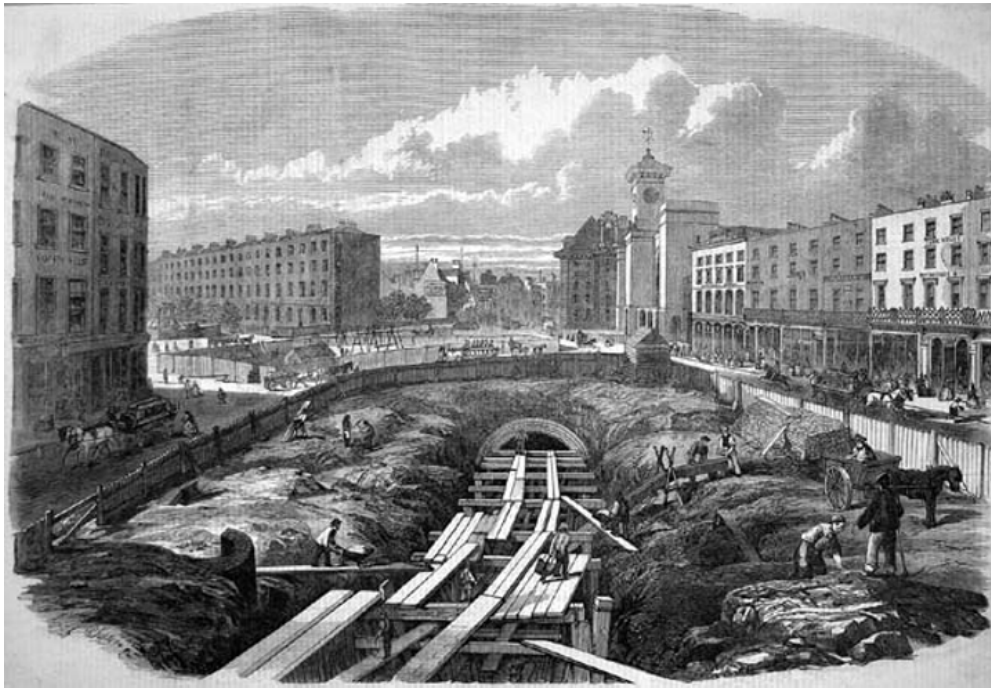
Figure 3. Construction of the world's first underground railway, the Metropolitan Line in London, 1861. Image freely available from Wikicommons at: http://en.wikipedia.org/wiki/File:Constructing_the_Metropolitan_Railway.png
